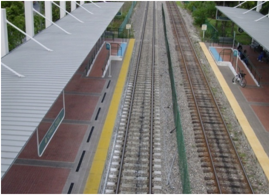
Figure 4.5 - Tactile Warning Surface at Platform End
