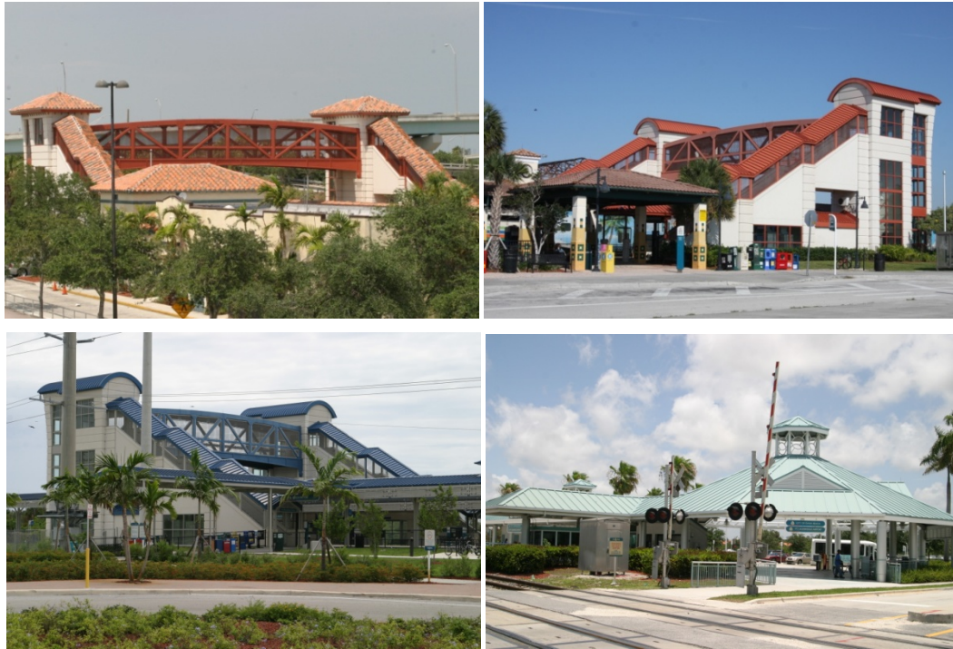
FIGURE 4.5 TYPICAL PLATFORM CANOPIES
